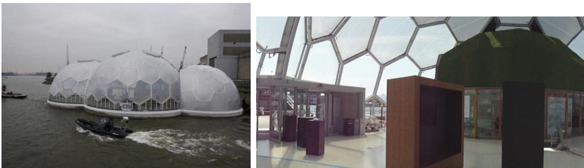
Ill. 2 and 3: Exterior and interior of floating pavilion 'De Zeebel', Inner harbor Rotterdam, 2010
