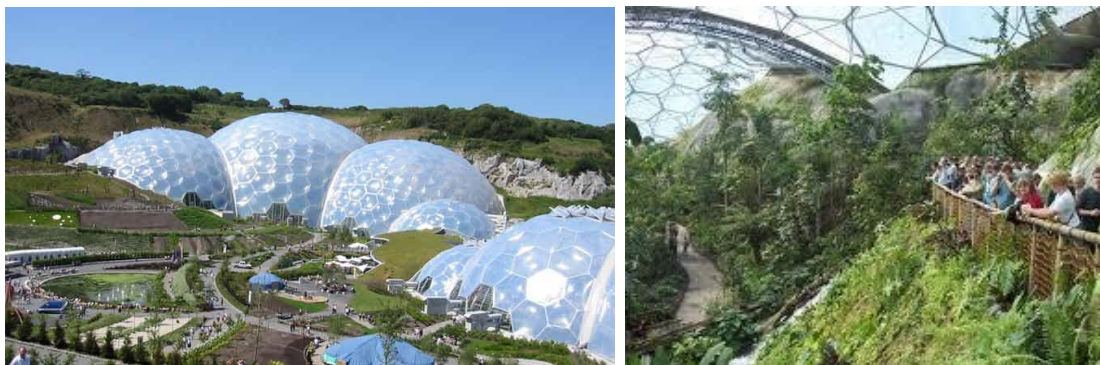
III. 6 and 7: Nicholas Grimshaw, Eden Project, Cornwall, view of outside and inside
